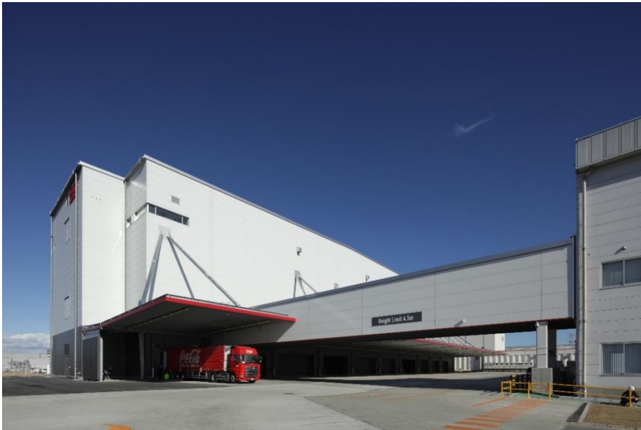
Exterior view of the Saitama Mega DC
